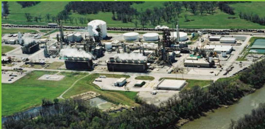
Terra Nitrogen plant in Verdigris, Oklahoma.
